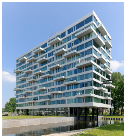
Abb. 48, Wiel Arets, Four Towers, Osdorp (NL)
